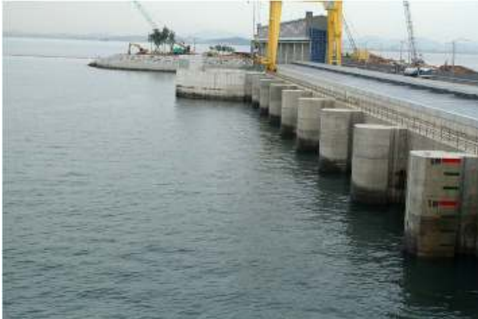
Figure: Sihwa Lake Tidal Power Station, located in Gyeonggi Province, South Korea, is the world's largest tidal power installation, with a total power output capacity of 254 MW.
