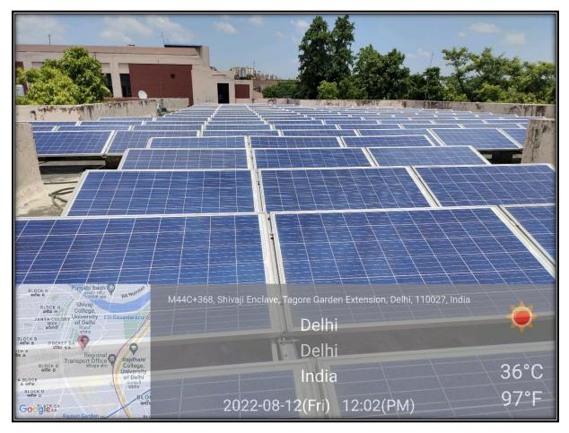
75 KWp roof-top solar panel installed by TATA Power on the roof of college for production of electricity. Excess power generated is transmitted back to the grid.
